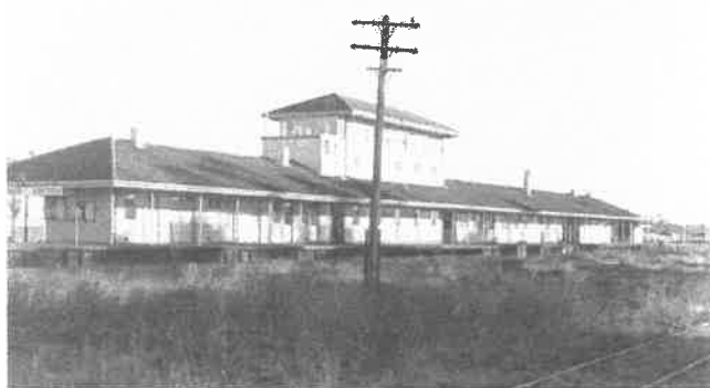
Railway Station with signal cabin upstairs
