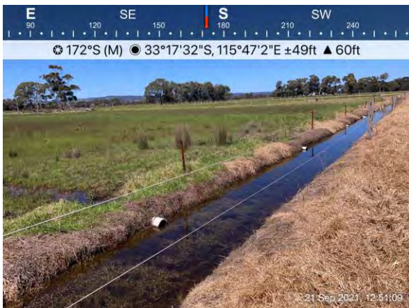
Photo 3: View to the south of open channel distribution network located in the north. The drains were historically used for irrigation via flood irrigation techniques. The drains at the time of the site investigation were filled with groundwater.
