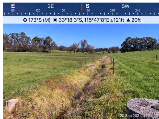
Photo 4: View to the south of cut drain in the southeast of the site. Cut drains in the Subject Site south of Treendale Road appear to be constructed for drainage of the site where as the drains in the north were constructed for historical flood irrigation use.
