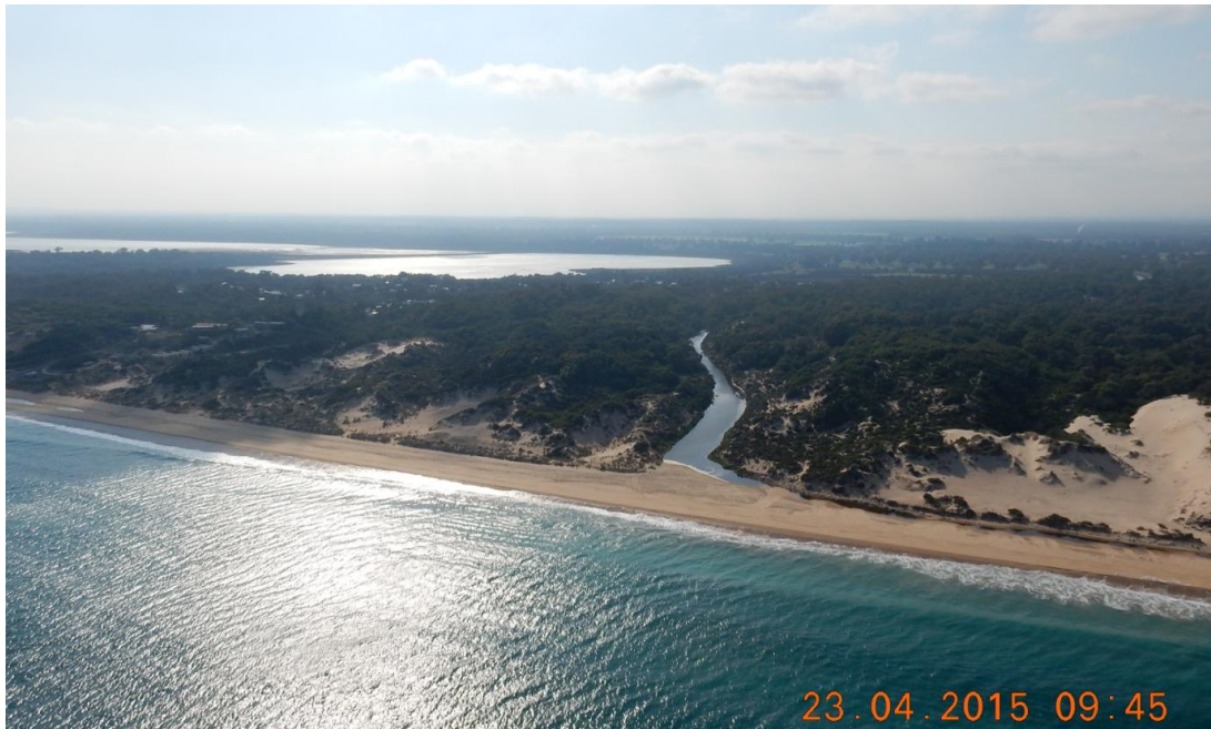
Figure 6-19: Harvey Diversion Drain Ocean Entrance Oblique View
