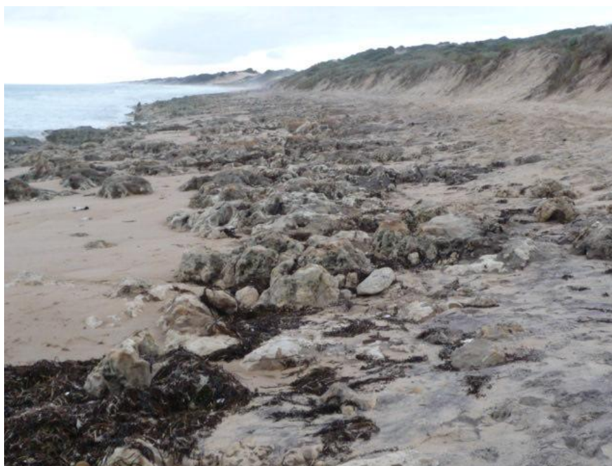
Figure 6-3: Exposed Beach Rock at Northern End of Binningup Town Site
