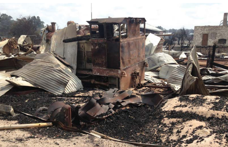
Post-fire remains of the historic Yarloop Railway Workshops. Photo courtesy of the Shire of Harvey
