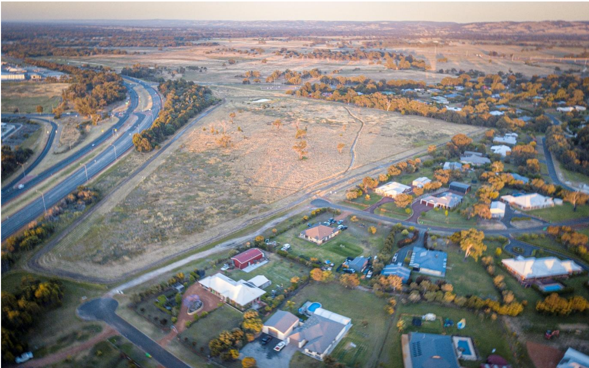
Aerial Photo Looking North Showing Existing MLRR Houses and Currently Vacant Lot 401
